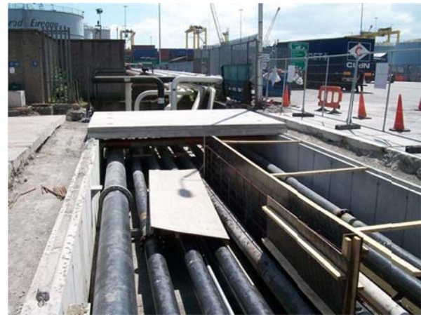
Figure 1. Oil pipelines exposed for maintenance (Photo credit: Eric Jones) [2]
